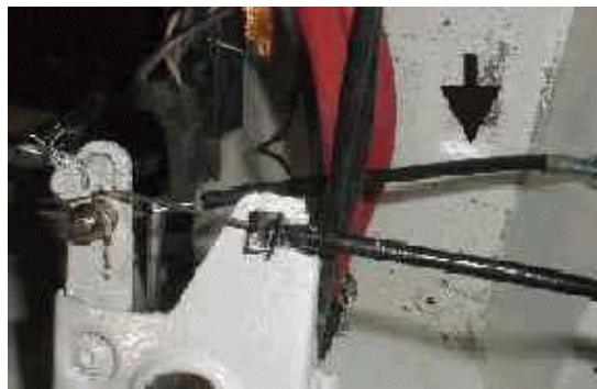
Figure 2. Supplementary hood release installed (the arrow shows the new cable).
