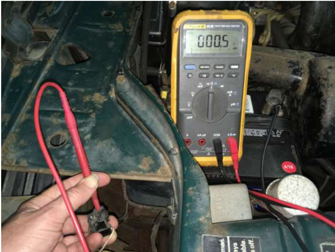
Verifying continuity to ground
